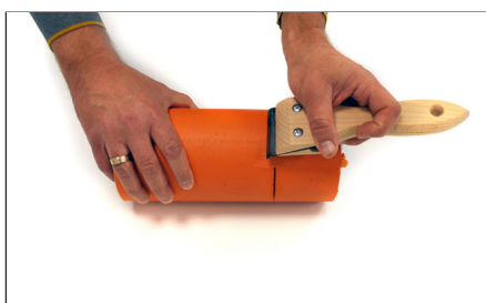
5. Gratter la zone de soudage du tube. Scrap the welding zone of the pipe.
