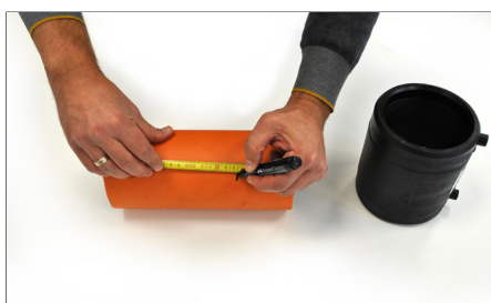
4. Mesurer la zone à gratter. Measure the scraping zone.
