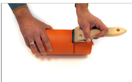
5. Gratter la zone de soudage du tube. Scrap the welding zone of the pipe.
